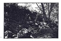
Cuttings and embankments are found mainly in the upper section. Many of the embankments are clad in dry stone walling many metres deep and can be seen from the road but many have been covered by the abundant vegetation. Some early dry stone walls can be seen on the upper bank of the road alongside more modern rock walls. One of the original stone embankment walls is found near the Sandy Creek Bridge
